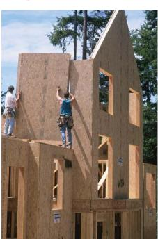
with stick framing. Builders may choose to build with SIP walls and a conventional truss roof, or stick walls and a SIP roof with little difficulty. SIPs are also popular as a method of providing a well-insulated building envelope for timber frame structures.
